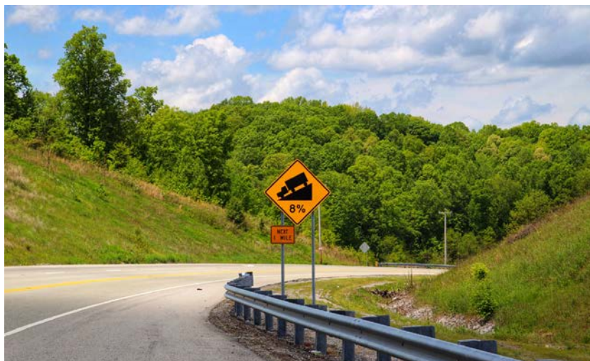
Figure 20. An 8% Grade roadside sign on S.R. 49 along the Tennessee River Trail in Houston County.
