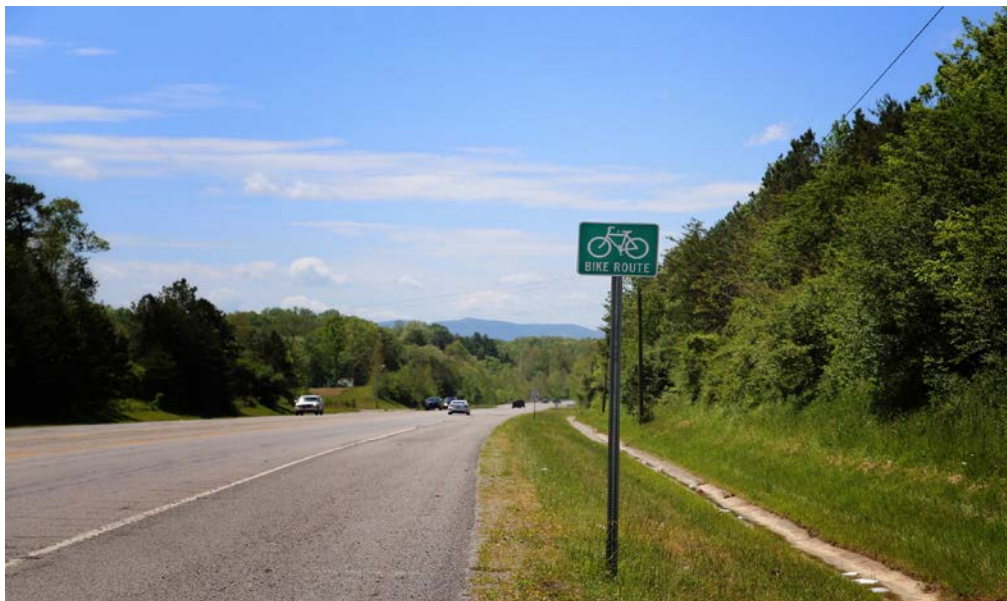
Figure 22. A Bike Route roadside sign and wide shoulder along a section of the East Tennessee Crossing National Scenic Byway (U.S. 25E) in Grainger County.
